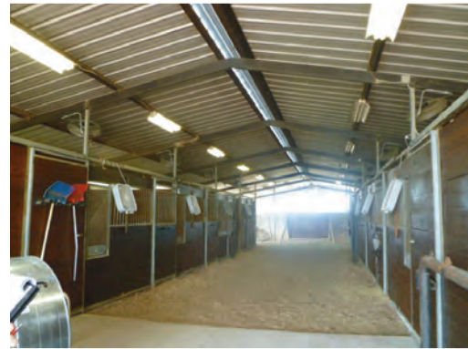
Modular stalls with swing out feeders, fans, insect system.
